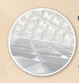
Approximately 11,000 quatrefoils line the glass of Christ Cathedral. Made of aluminum, the triangle-shaped panels are perforated to allow for sunlight, while also deflecting ultraviolet rays and heat from the glass. The quatrefoils have a polycarbonate backing and fiber to improve acoustics for the Hazel Wright Organ, as well as
